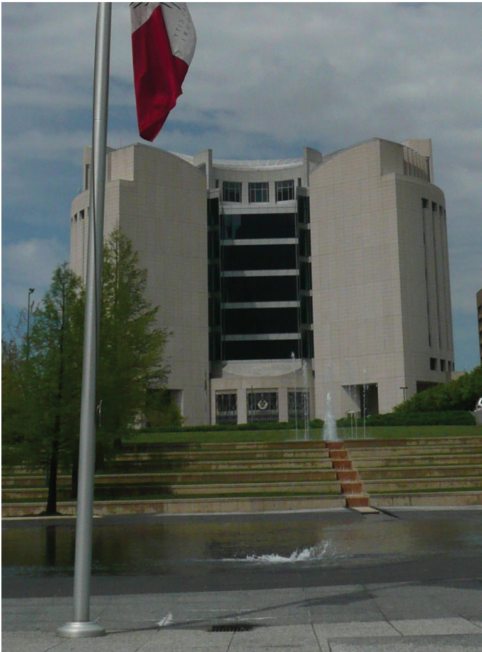
Figure 4. Whittaker Federal Building, Kansas City, MO (1998)
