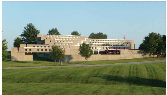
Figure 2. Clay County Annex, Kansas City, MO (1980)
